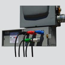
without the need for an electrician. Installed at the base of an existing manual disconnect switch. transfer switch, or main circuit breaker panel, these cost-effective panels help building owners integrate portable generators or load banks into their electrical systems for reliable and uninterrupted power performance in any scenario.
