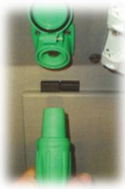
Insert Cam-Lok fully into the receptacle.
