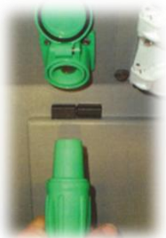
Insert Cam-Lok fully into the receptacle.
