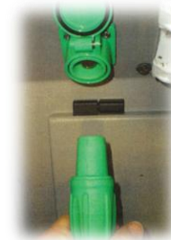
Pull Cam-Lok connector straight out of the receptacle; do not twist or force.
